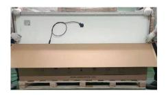
Two workers take out the module from the box. Then repeat step 5 and 6 to take out the other modules one by one.
