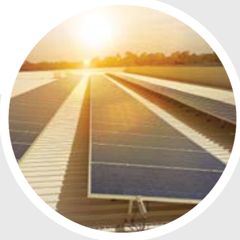
2. IKEA NATIONAL PROJECT, VIC, NSW & QLD Module: CS6X-P and CS6P-P Power generation: 3.6 MW
