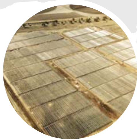
6. OAKLEY SOLAR FARM, QLD Module: CS6U-M, CS3U-P Power generation: 100 MW
