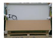
Two workers take out the module from the box. Then repeat step 5 and 6 to take out the other modules one by one.
